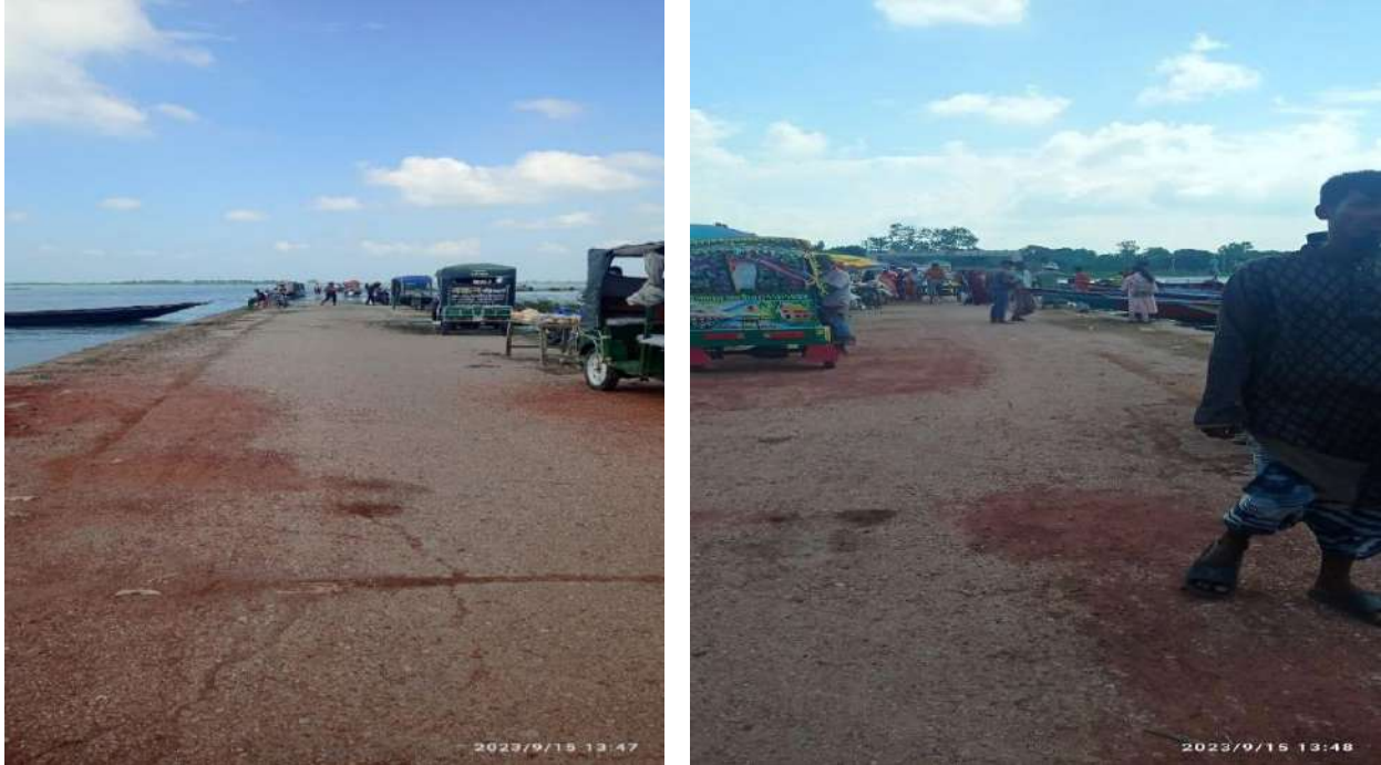
Figure 10: Existing Condition of Roads (Source: Field Survey, 2023)
