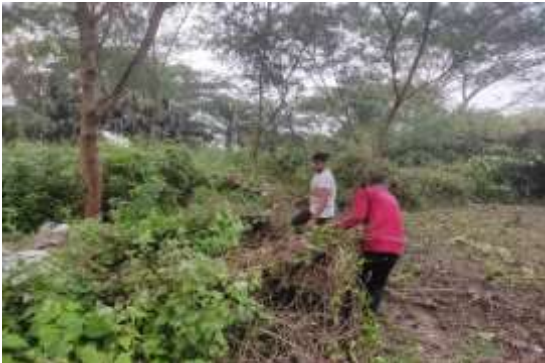
Figure 4: Cleaning the Acquired land
