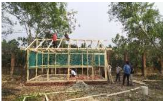
Figure 1: Building House to Accommodate the Compost Plant
