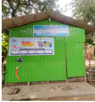
Installation of water treatment plants
