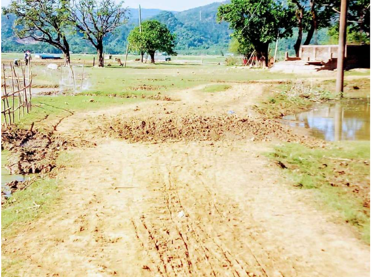
Photo: Muddy roads in Indrapur Village, North Sreepur Union (Credit: Author)
