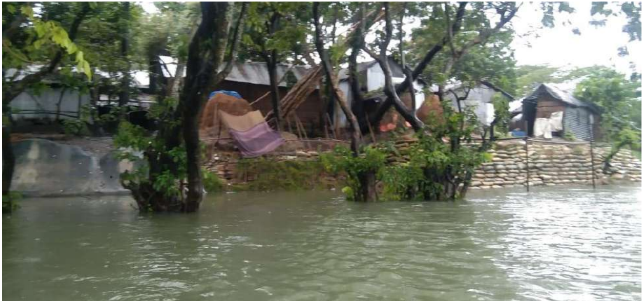
Photo: Earthen Embankment in Janjail village, South Sreepur Union (Credit: Author)
